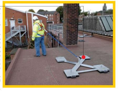
faces, including single-ply membrane, asphalt, concrete, stone chippings (brushed), and mineral felt. The metal components are galvanized to BS EN ISO 1461 for corrosion resistance and long life.
