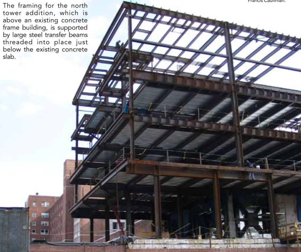
The framing for the north tower addition, which is above an existing concrete frame building, is supported by large steel transfer beams threaded into place just below the existing concrete slab.
