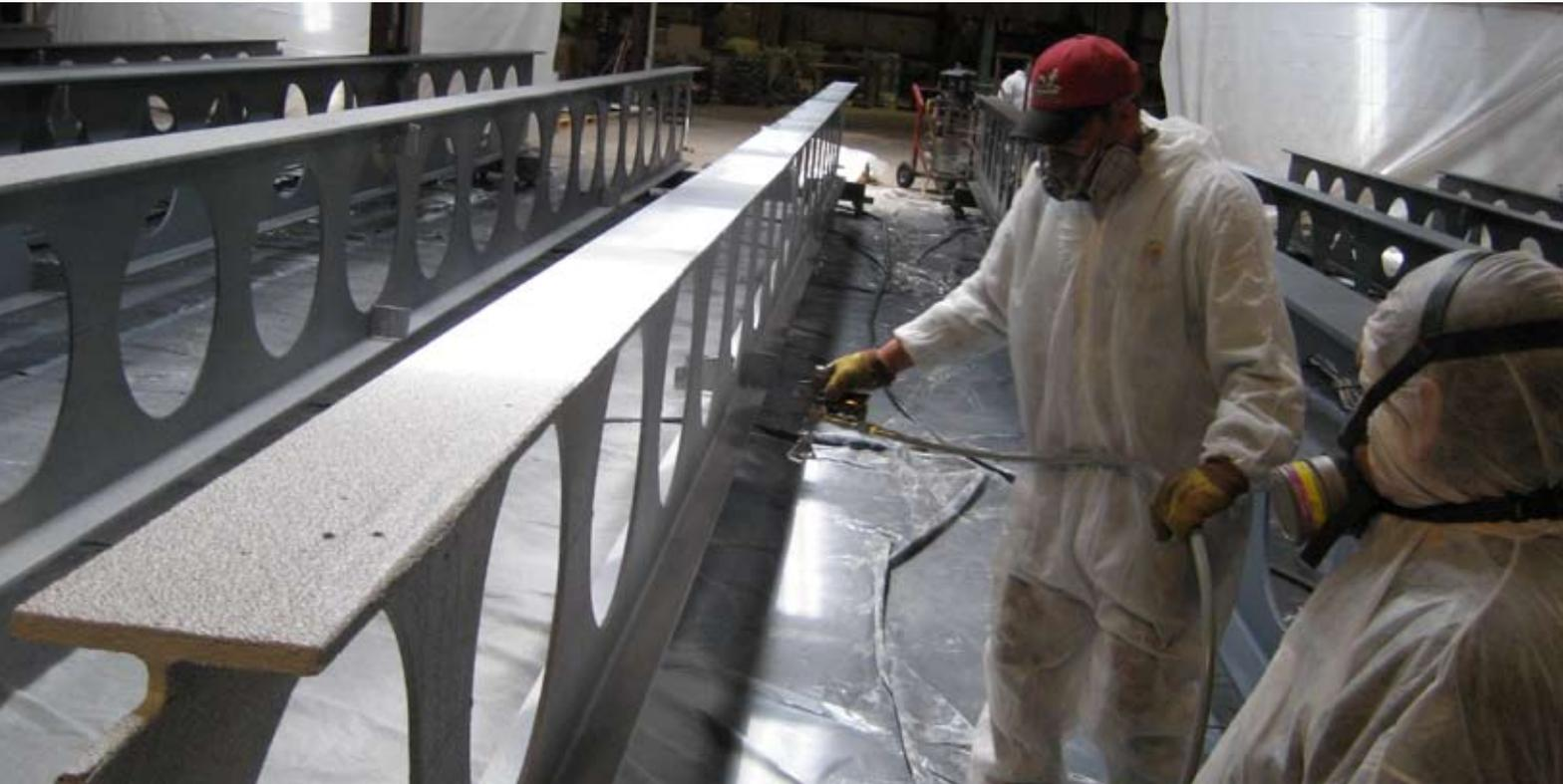
**Above:** A fireproofing system consisting of primer, a layer of carbon fiberglass mesh between two layers of intumescent fireproofing material, and a polyurethane topcoat was applied at ground level and in a climate-controlled environment in the fireproofing contractor's facility.
