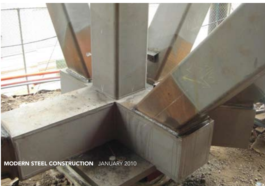
Below: The HSS braces were bolted to the underside of the first floor beams and landed directly onto the column base boxes at the bottom with full-depth partial penetration welds.
