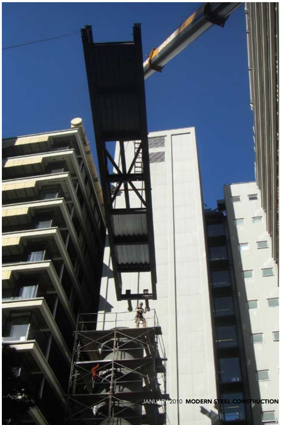
Below: The first of two sections of the access bridge floor framing being hoisted into place, from the mechanical yard 90 ft below, shows the tight clearances to the existing Health Science Building, where it connects the ninth floor with the main entrance of the new Regeneration Medicine Building.
