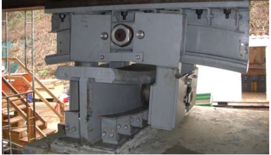
Above: The unique uplift restraint devices installed in eight locations along the uphill line of supports were fabricated as part of the structural steel fabrication.
