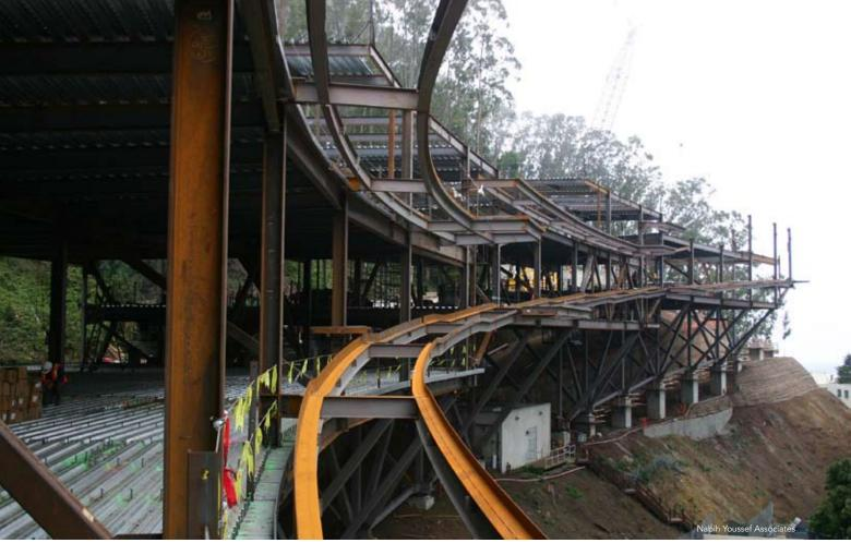
The RMB under construction by DPR Construction and Schuff Steel. Steel framing for the cantilevered walkways is clearly visible here, as is the existing fire pump building over which the new structure is being constructed.
