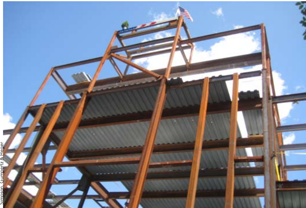
Photo of the front elevation during construction showing the exposed secondary steel girt structure which supports the veneer. The steel columns closely match the depth of the steps and the steel beams frame to either the inner or outer flange.
