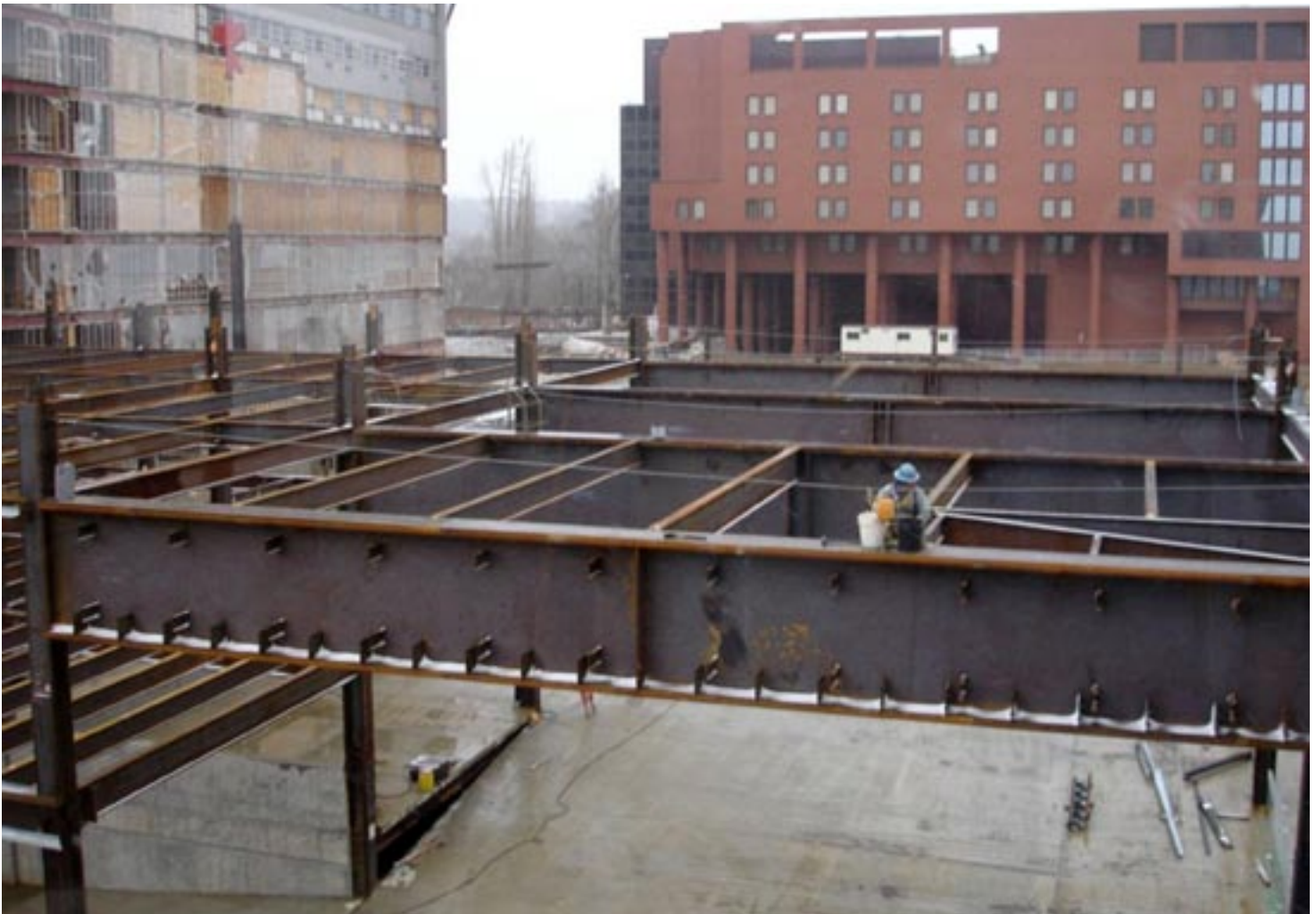
Opposite page: Building a new 13-story hospital on a century-old medical campus in Pittsburgh's Lawrenceville section presented both opportunities for renewed vitality and the challenge of working in tight quarters.
