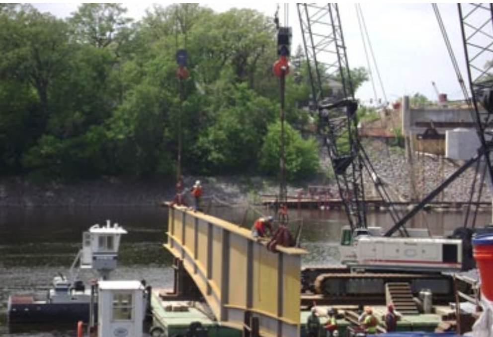
left, top: The haunched section of this interior girder shows the longitudinal stiffeners that were required at the river piers.
