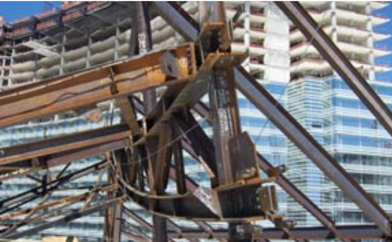
Extra tabs and attachment points had to be provided for the variety of cables that stabilized structural elements throughout the steel erection.
