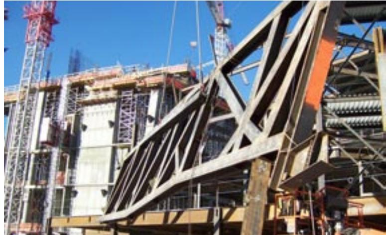
Lifting devices engineered to allow the crane to hold members at the proper skew and slope reduced the brute force required of the ironworkers in making connections.
