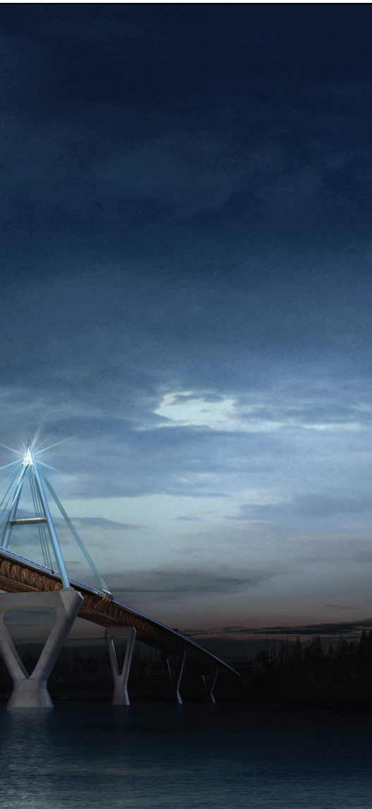
The Deh Cho bridge will provide a year-round means for crossing the Mackenzie River in Canada's Northwest Territories where until now access has been seasonally interrupted.
