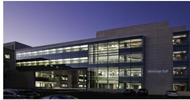
**Above**: A 14-ft cantilever beyond the truss structure provides additional office space on this bridge on the campus of Northwestern University.
