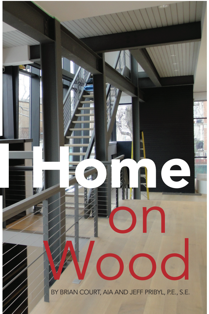
This page: Three views of the main floor with the main steel moment frame running the length of the house.
