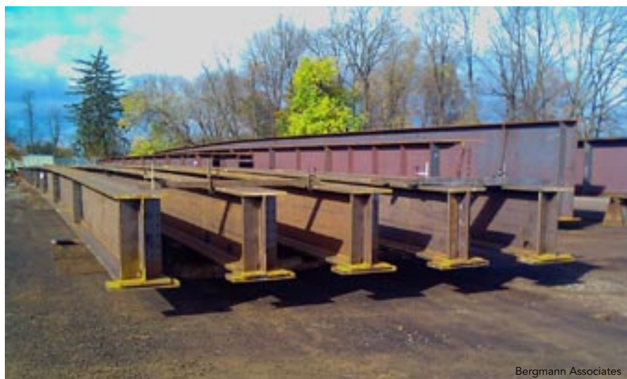
Steel plate girders for the replacement 9 Mile Road bridge over I-75 were delivered to the contractor's staging area for quick job site deployment and erection when the piers were completed.
