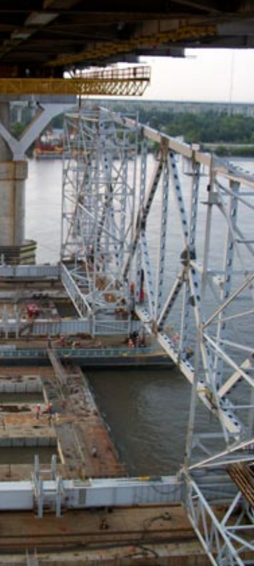
Fig. 7: Horizontal jack slides sled-mounted strand jack 13 feet, carrying truss panel over its bearing.
