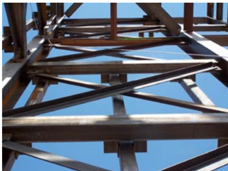
▲ Full-height cross-braces at the corners provide stability to the Urban Lantern tower.
