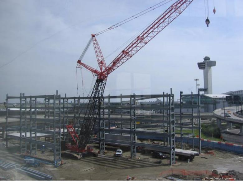
As part of constructing the new Terminal 5 at New York's John F. Kennedy International Airport, the Port Authority of New York and New Jersey added a steel-framed new six-story parking structure for 1,500 cars. ▲ The design-build team's decision to use steel framing with longspan precast spandrels resulted in an open parking structure and reduced both the initial cost and maintenance requirements.
