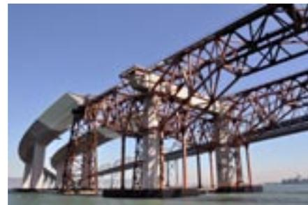
▲ **Build.** Taken on a recent field trip to the new San Francisco-Oakland Bay Bridge, this photo shows the scale of temporary steel trusses wrapped around the reinforced concrete bridge piers. The trusses will support the white steel box girder bridge deck of the self-anchored suspension bridge during construction.
