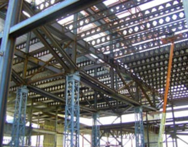
◀ Three catenary trusses support the majority of the floors above the exhibit hall, with an arch truss at the end of the building where the catenary would have extended outside the building.
