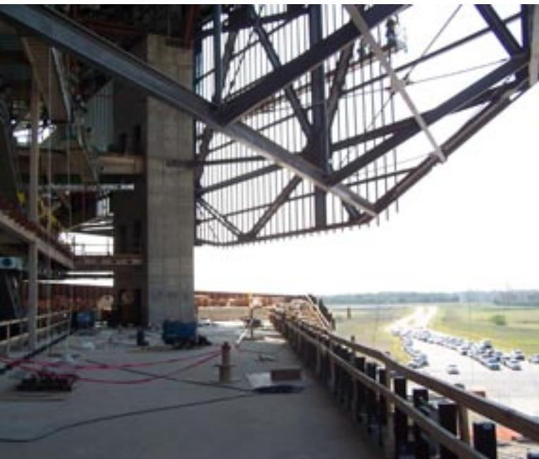
▲ The concrete elevator core provides a fifth support point on the south side of the structure, reducing the required truss span from 300 ft to just 190 ft.
