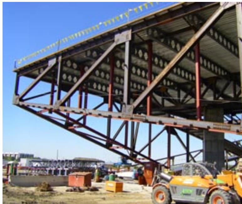
▲ Cantilevering the floor structure over the two main entries allowed the area to remain column-free.
