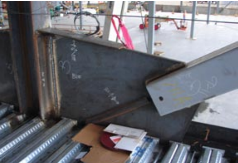
DETAIL AT WF COLUMN WEB CONDITION
