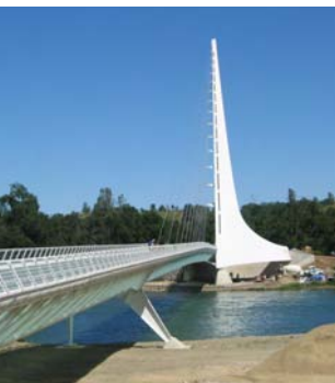
2004: Santiago Calatrava's Sun Dial Bridge in Redding, Calif., works as both a sculpture and as a bridge.
