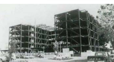
1980: The O'Connor Hospital in San Jose, Calif., is an early use of eccentric braced frames for seismic design.
