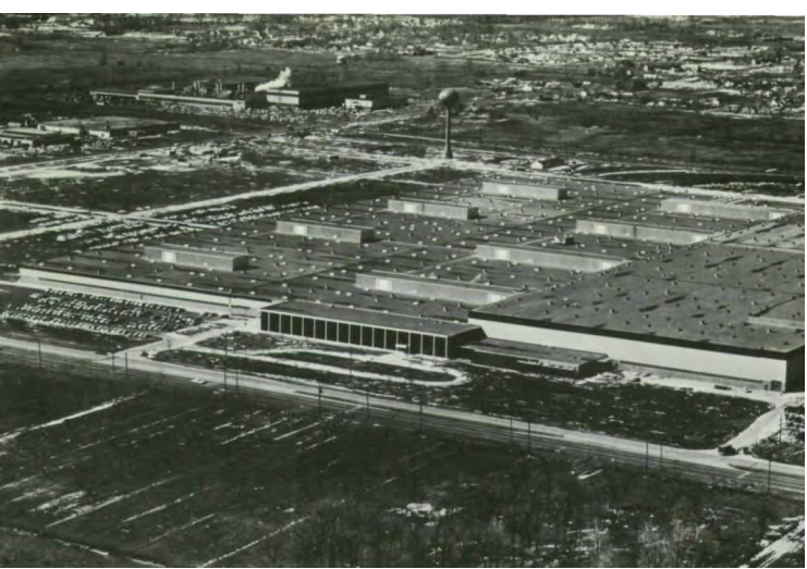
1967: Setting what might be a record for a building of its size, a 2.6-million-sq.-ft Chrysler plant was designed and constructed in just 11 months.
