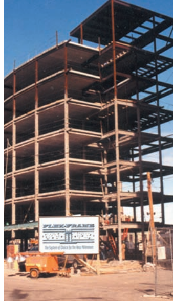
2000: A new system using concrete plank atop a grid of asymmetric steel members is used on a new Drexel University dormitory building. The result is low-floor-to-floor heights and incredibly rapid construction. The system ultimately leads to the development of the increasingly popular Girder-Slab® System.
