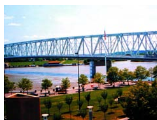
1997: Combining Grades 70W, 50 and 36 on the Central Bridge between Newport, Ky., and Cincinnati allowed the designers to maintain a constant girder depth.
