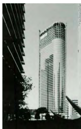
1983: Four Allen Center in Houston is designed as a circue-ovular building to reduce wind loads.
