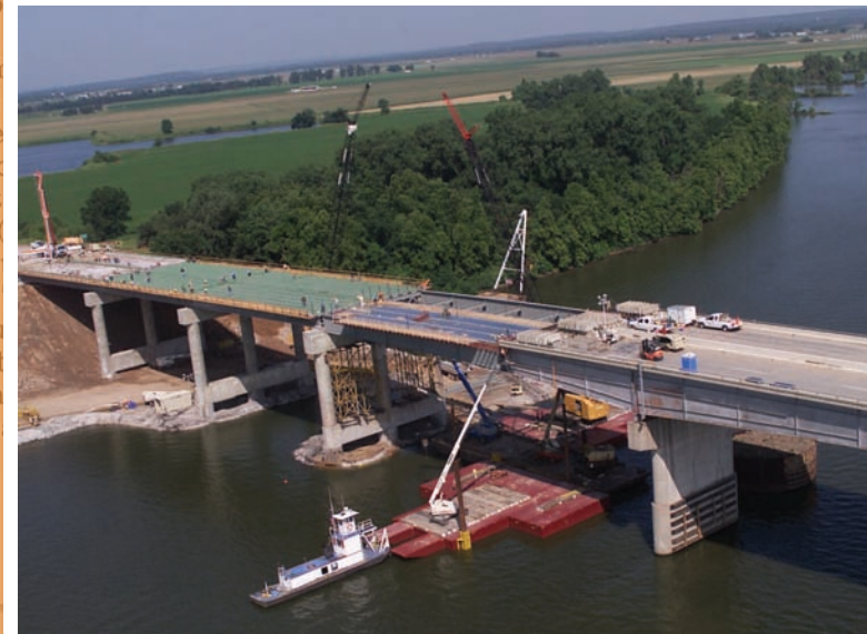
2002: After a pair of errant barges knocked down the I-40 bridge at Weber Falls in Oklahoma, the steel industry mobilized to get a new bridge up and open in just two months.
