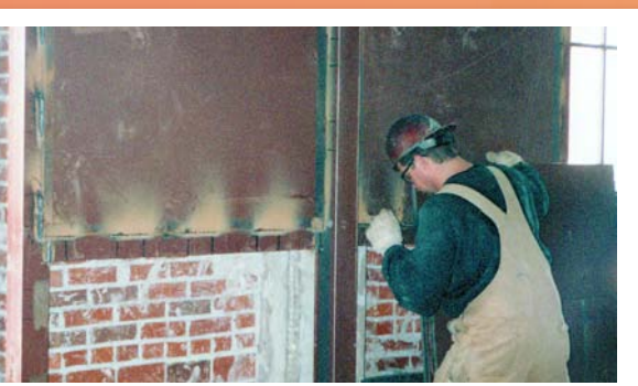
2000: The steel-plate shear wall installed during the rehabilitation of the Oregon State Library in Salem was a precursor to a system that gained popularity later in the decade.
