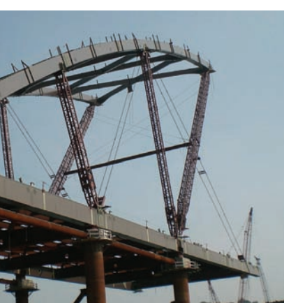
2007: The Blennerhassett Bridge over the Ohio River between West Virginia and Ohio used 30 million lbs. of HPS for its 4,000-ft span.
