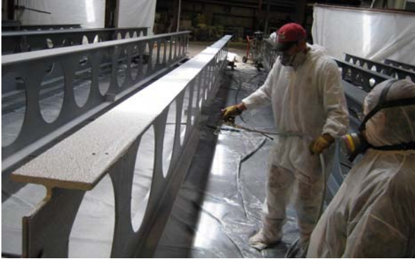
2009: Shop-applied intumescent fire protection cuts the construction schedule on the the BJC Institute of Health in St. Louis.
