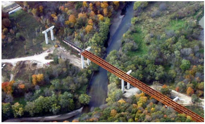
2004: The US20 bridge over the Iowa River is the first in the U.S. to use the incremental launch method for erecting an I-girder bridge.
