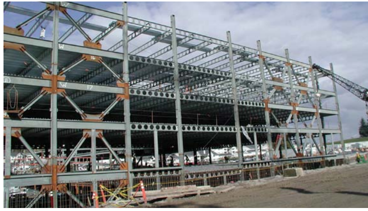
2005: The parking structure for the Legacy Salmon Creek Hospital in Vancouver, Wash., is an early example of the SmartBeam™ system in a parking structure.
