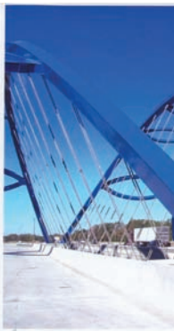
2007: The Gateway Bridges on I-94 near Detroit mark the first time tied arches are built with longitudinal ties buried under the road. The innovative system solves the redundancy issue with tied arches.
