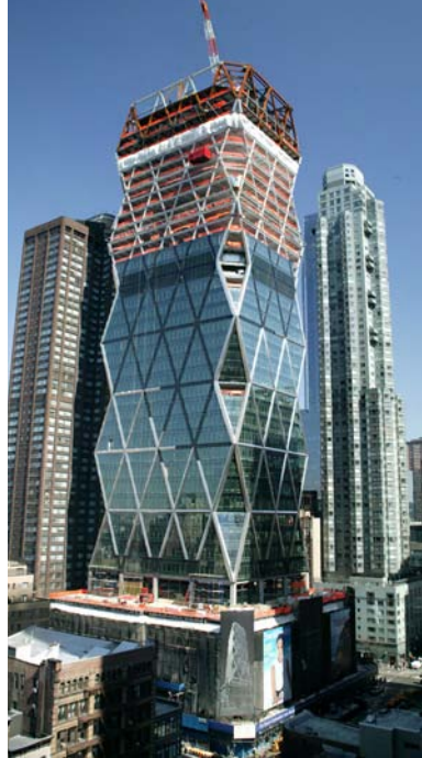
2006: A diagrid steel frame gained attention for the 46-story Hearst Building in New York City.
