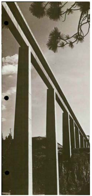
1973: The Latah Creek Canyon Bridge in Spokane is an early example of a steel box girder bridge.
