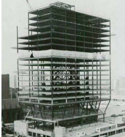
1981: One Corporate Center in Hartford, Conn., demonstrates the growing trend toward vertical expansions as it rises 16 stories on top of an existing building.
