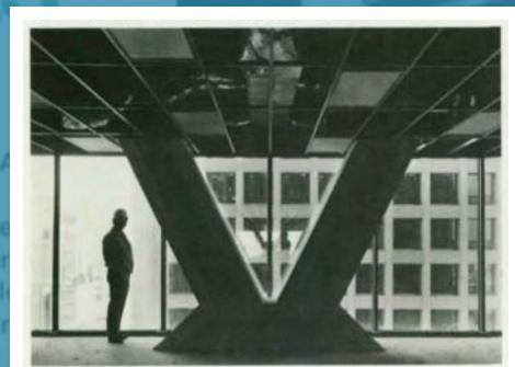
1976: The 56-story First International office building in Dallas features a trussed tube design with diagonal X-bracing and stub girders.
