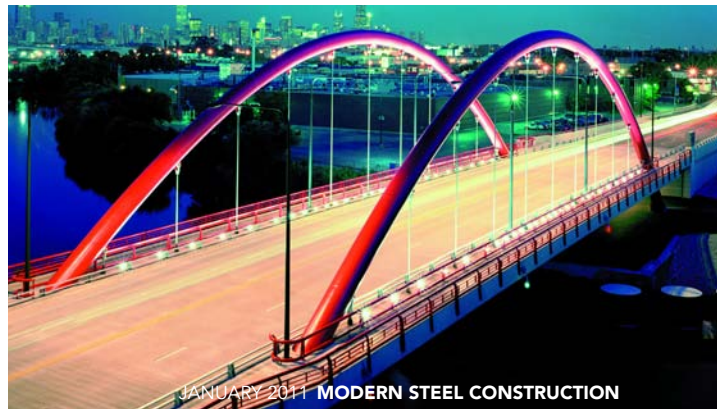
1999: Damen Ave. arch creates a new neighborhood landmark in Chicago while also demonstrating the economy and speed of construction of steel.
