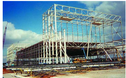
1999: It only took 26 months from the start of design to the completion of construction on the 1.5-million-sq.-ft Boeing Rocket Booster facility in Decatur, Ga.
