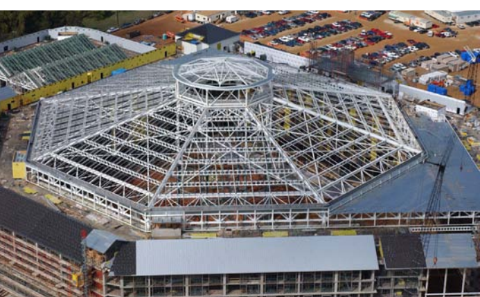
2003: The Gaylord Texan featured cellular steel beams—and will play host to NASCC: The Steel Conference in 2012.
