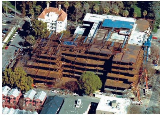
2003: Steel framing dominates the early ranks of LEED-certified buildings, including one of the first Gold projects, the Department of Education Building in Sacramento.
