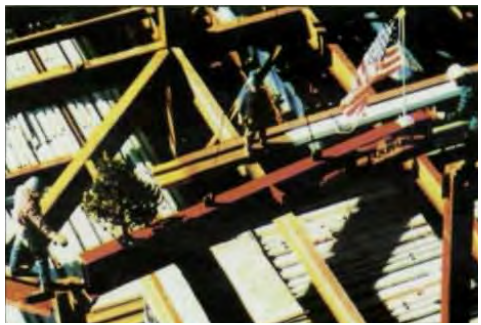
1995: Finally answering the question of why we put a Christmas tree atop a building during the topping out ceremony.
