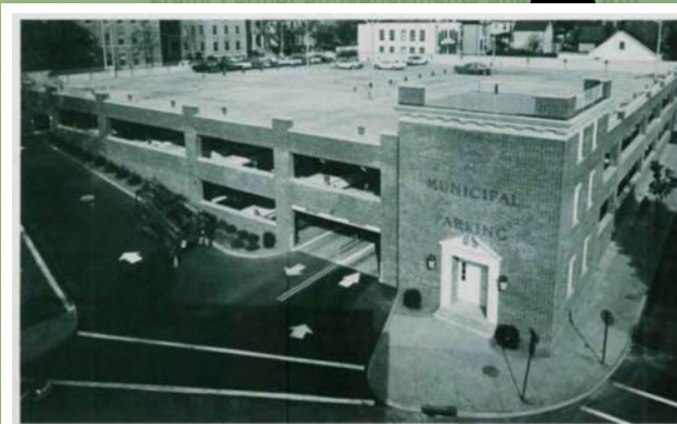
1963: Parking structures were a growing market and AISC showcased several projects using high-strength steel to minimize columns and reduce costs.
