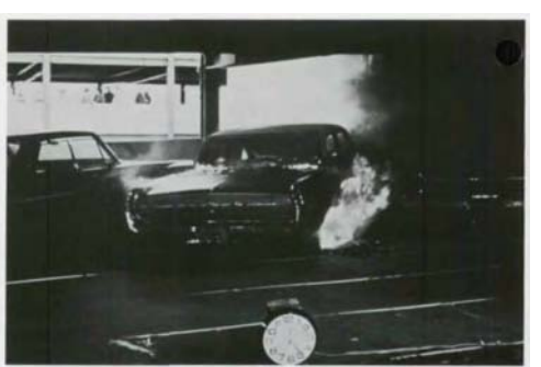
1973: The first coverage of AISI's Scranton fire tests, which demonstrate that fire protection is not needed in open-air steel parking structures.
