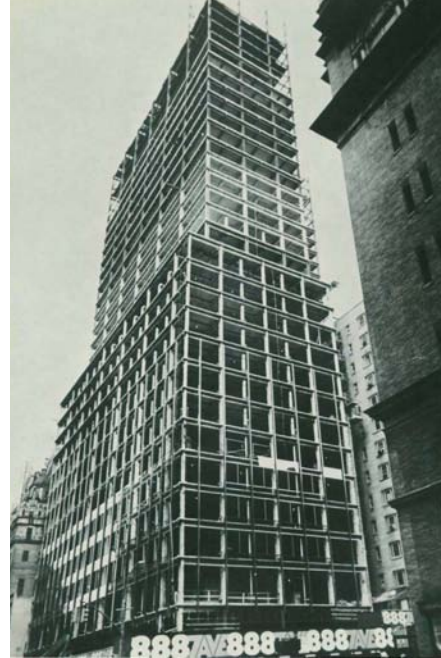
1969: 888 7th Ave. in New York is an early use of composite construction.
