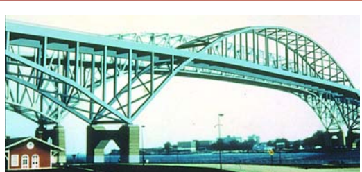
1997: The Blue Water Bridge between Port Huron, Mich., and Sarnia, Ontario, is an early example of the use of LRFD in bridges (it was also designed with all SI units).
