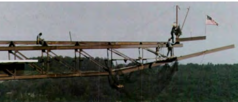
1988: A tube of wide flange sections creates an "infinity room" and a new tourist attraction at the House on the Rock in Spring Green, Wis.
