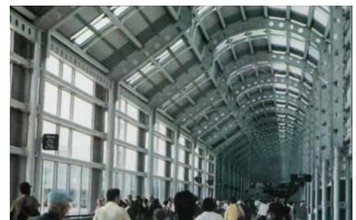
1987: The United Airlines terminal in Chicago helped popularize both the use of curved steel tubes and exposed structural steel.
