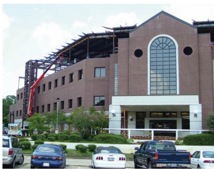
2008: Southpark Hospital in Shreveport, La., remained fully operational while an additional floor was added.
