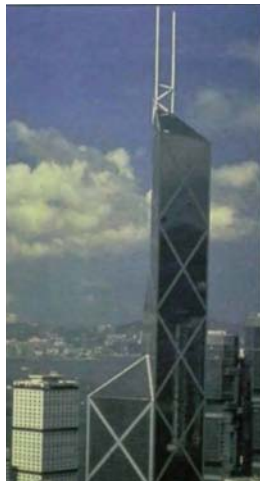
1994: Larry Griffis' T.R. Higgins lecture offered everything you need to know about composite frame construction, using the Bank of China in Hong Kong as one example.
