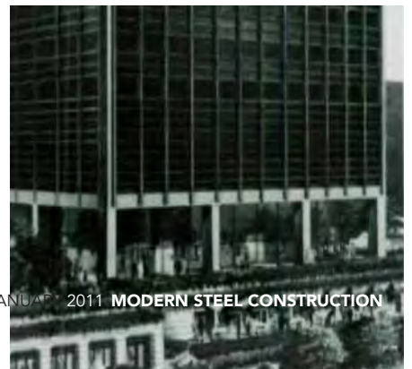
1987: The Quaker Tower in Chicago uses its central core as its complete lateral load resisting system.
