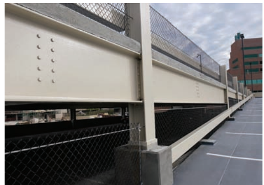
2008: A steel framed, post-tensioned slab system proved economical for a parking structure at Ruby Memorial Hospital in Morgantown, W.Va.
