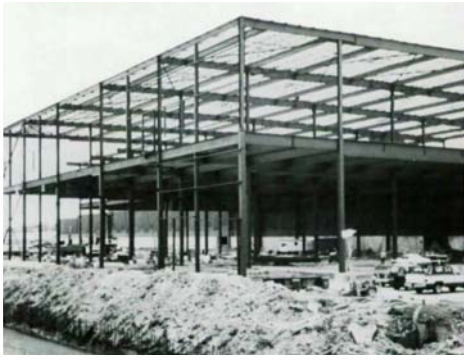
1985: Fast track construction is all the rage; the 172,000-sq-ft Federal Express storage facility in Memphis goes from ground breaking to occupancy in just nine months.
