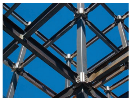
2005: Building 1 at Santa Row in San Jose, Calif., was one of the first to use the proprietary ConXtech system.
