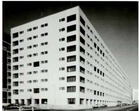
1983: The Barnes Building Rehabilitation team touts their extensive use of computer analysis using STAAD-III.
