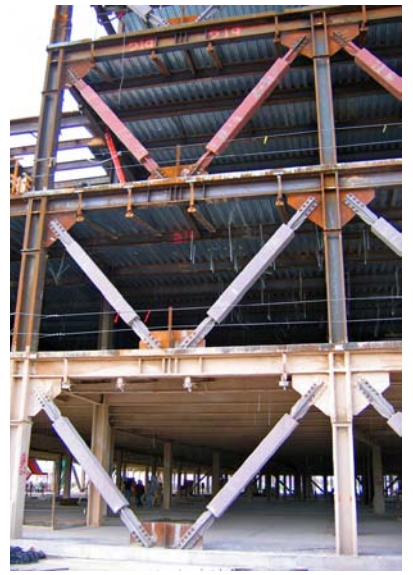
2005: Buckling Restrained Braced Frames (BRBF) became very popular later in the decade. Shown is an early example at the Intermountain Medical Center in Murray, Utah.
