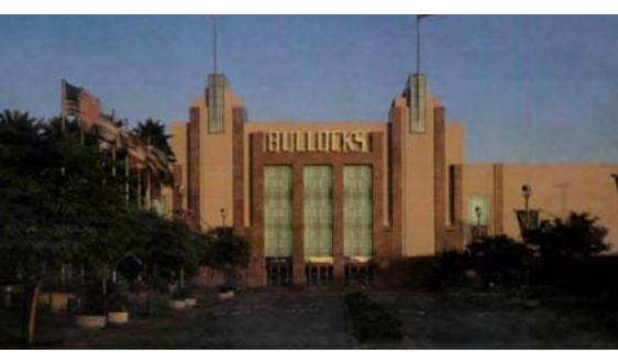
1994: Moment connections provided both long spans and structural stability on the Bullocks department store building in Burbank, Calif.
