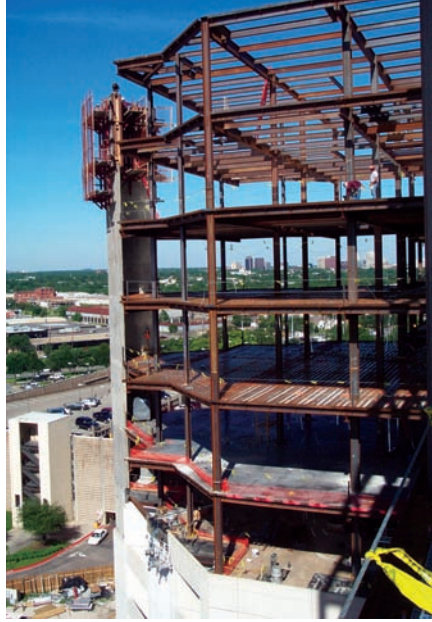
2003: For the Dallas Children's Medical Center, steel was the answer for adding six stories to the existing concrete structure.
