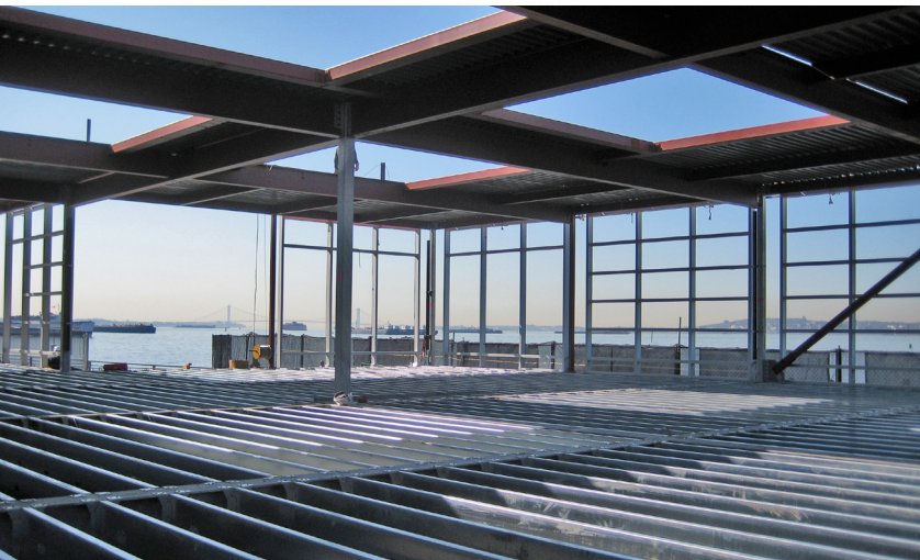
▼ The floor is supported by light-gauge steel studs spanning between W24 galvanized steel girders.
