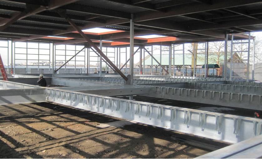
▼ The floor is supported by light-gauge steel studs spanning between W24 galvanized steel girders.
