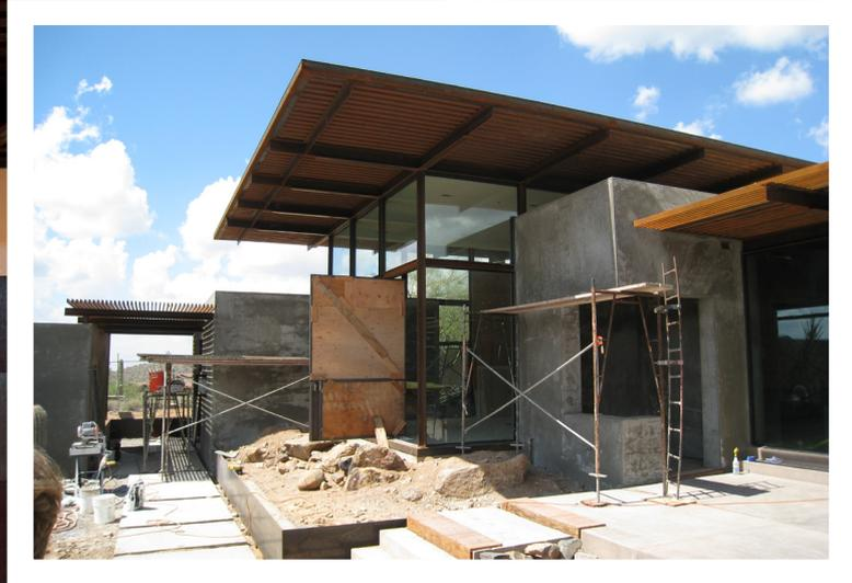
**Above, left, and below:** Using a uniform, simple, light steel framework of W4 columns and W8 beams provided the necessary structural support while minimized visual obstruction.
