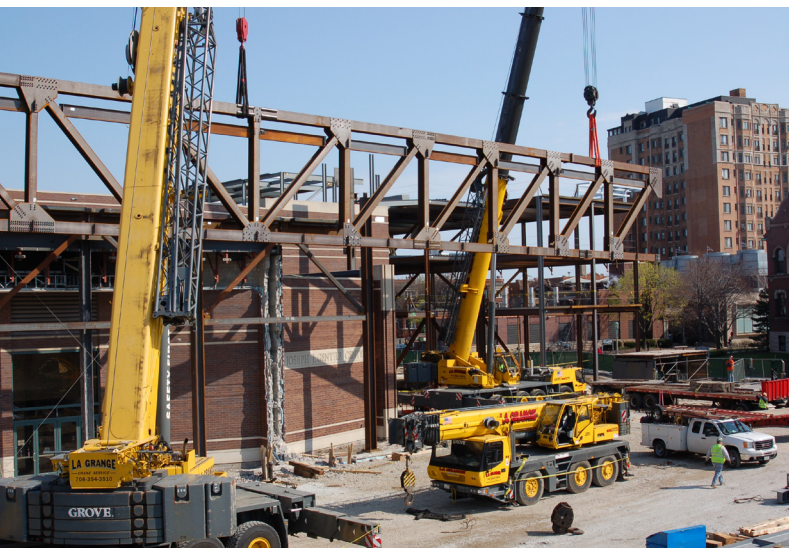
▲ The truss being lifted into place. Orienting the member webs perpendicular to the plane of the truss greatly simplified the field-bolted connections.
