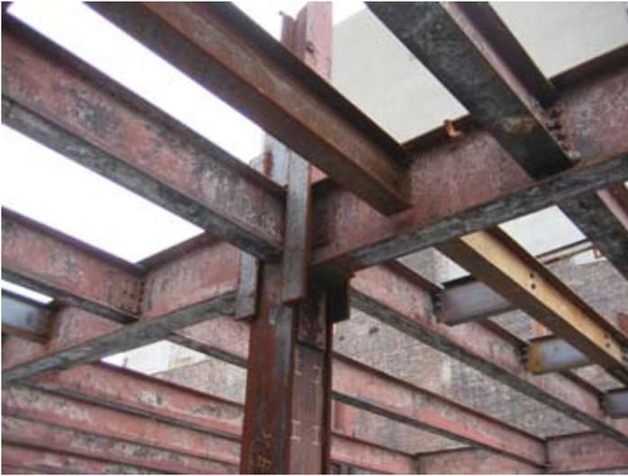
▲ Most of the warehouse's original steel framing remained in place for the new, taller, repurposed structure. Some concrete floor slabs were removed before raising the superstructure to lighten the dead load and facilitate the foundation upgrade.
