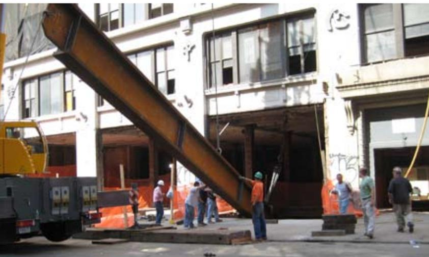
▲ One of four 44-in.-deep, 50-ksi built-up steel plate girders with 3/2-in.-thick flanges being lowered into the basement. The girders transferred column loads of as much as 900 kips and facilitated a foundation replacement under existing columns.
