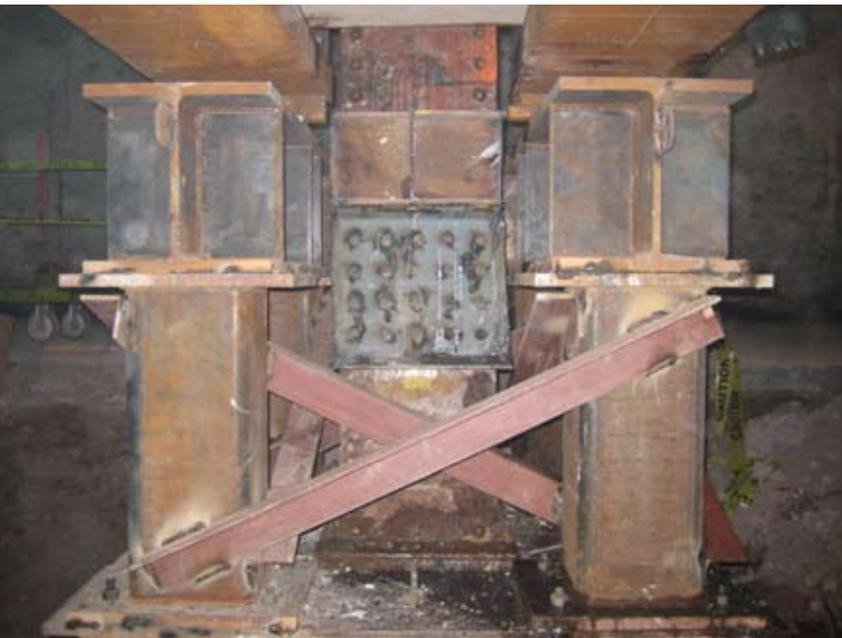
◀ Steel bearing pedestals ensured the redistributed and transferred loads were properly induced into the outer columns and footing system.
