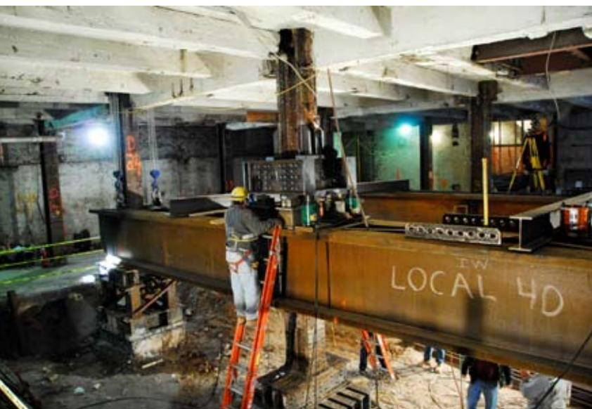
◀ The jacking process required four 150-ton hydraulic jacks for each steel collar and raised each of the four inner columns approximately 3/16 in.
