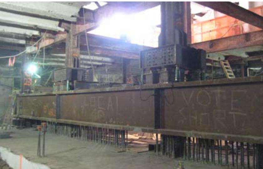
▲ The new 7-ft-thick mat foundation for the elevator core, constructed under the transfer beams, prior to infill placement. Once complete the column loads were transferred to the new foundation.
