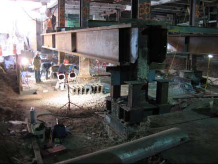
◀ Installing large transfer girders allowed portions of the existing building's strip footing foundation system to be severed, demolished, and removed to allow the new elevators to extend further below grade and through the existing footing supports.
