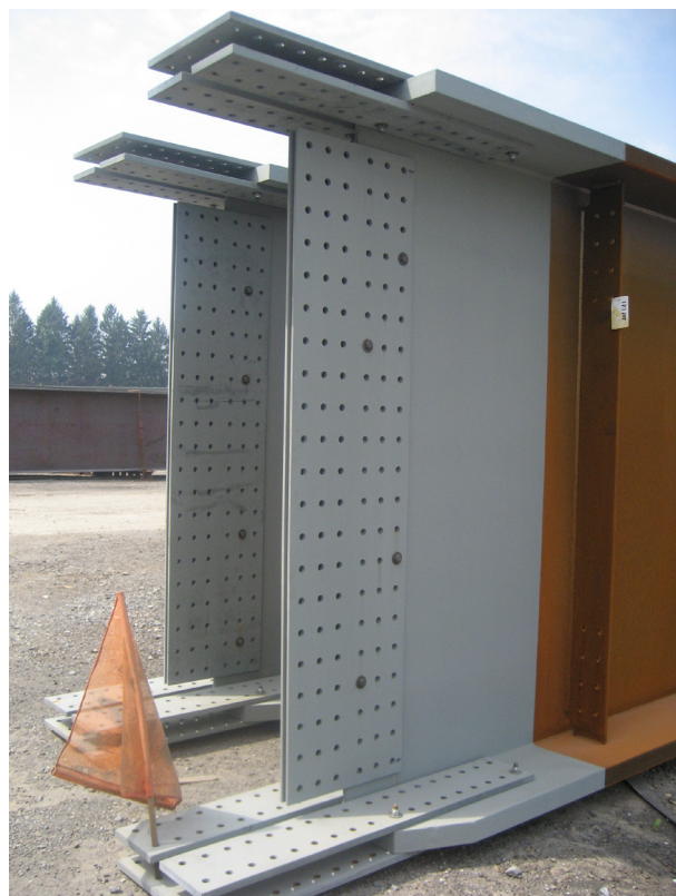
▲ This photo provides an example of two popular corrosion protection systems—painting and the use of weathering steel.
