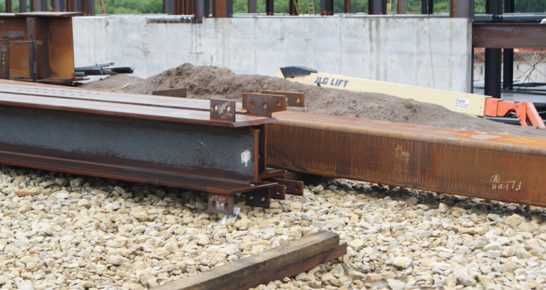
▲ Steel columns on site awaiting erection.
