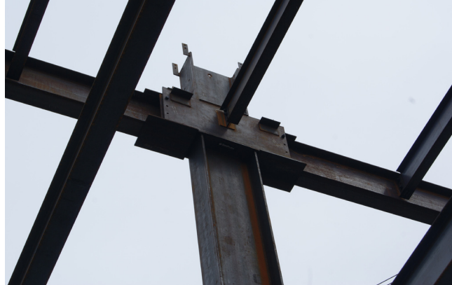
▲ SidePlate moment frame tree in the process of being erected.
