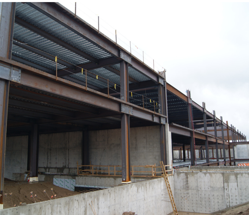
▲ View of hospital construction from the central energy plant.
