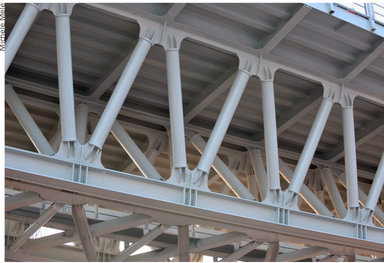
▲ Detail of the reticular spatial structure that successfully combines a lean look with solid seismic resistance.
