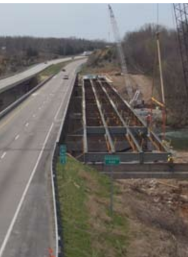
▼ Completion of steel erection.
