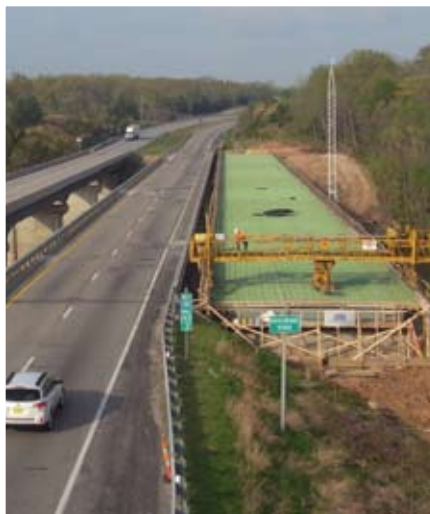
▼ Deck reinforcing complete and ready for concrete placement.
