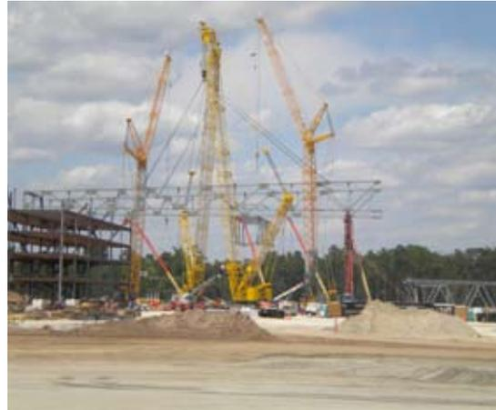
▲ The 610-ft-long trusses were assembled on the ground in two sections.
