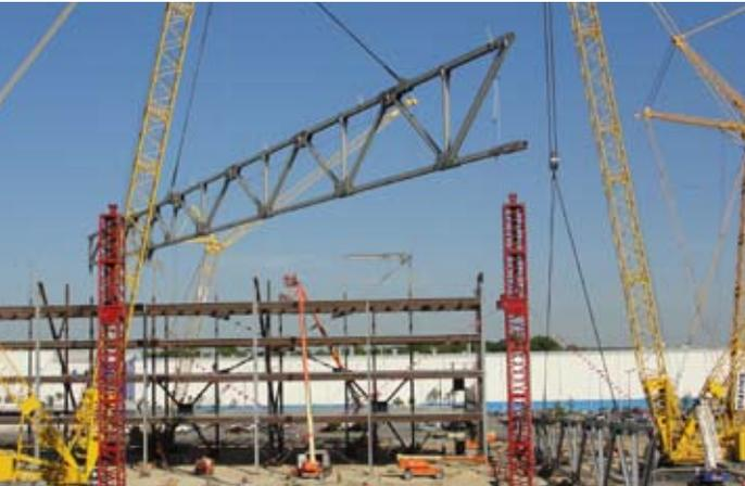
▲ As each section of the main truss was lifted, it had to be swung into the proper alignment perpendicular to the side buildings. The first two trusses were placed using a single falsework tower for each, as the side building provided support for the outer end.
