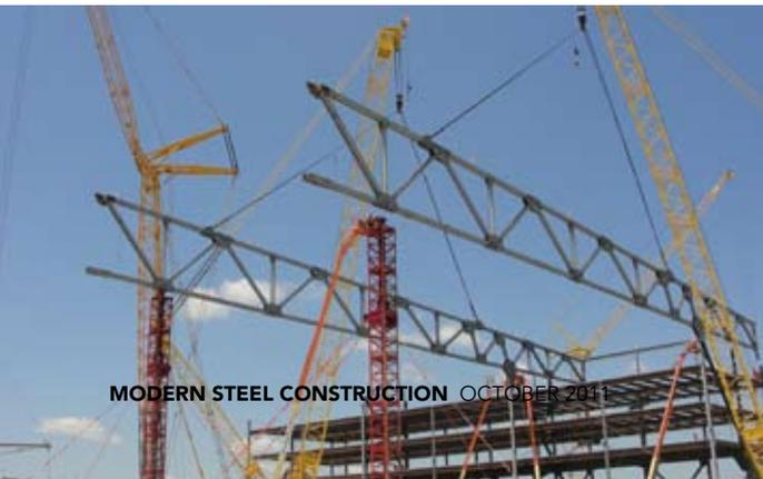
also designed to support 12 underhung moveable crane bridges, with three four-hook cranes that can be coordinated for lifts involving multiple cranes when necessary. CMC engineers used innovative design concepts in order to minimize the quantity of costly slip-critical connections, many of which required 300 1½-in.-diameter A490 bolts.
