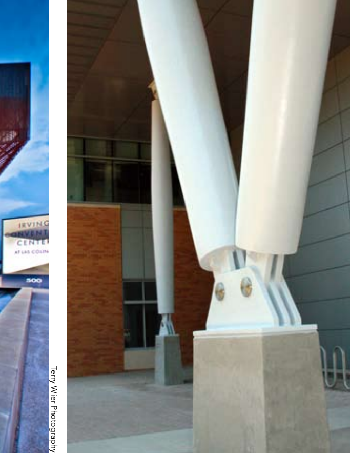
▲ Connections of built-up steel columns at the UNT Business Leadership Building had to be adjusted to account for the thickness of intumescent paint.
