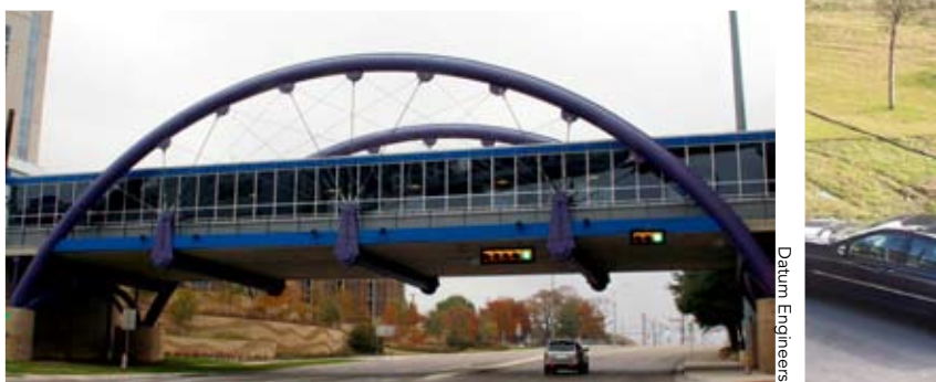
▲ The Children's Medical Center bridge features crisscrossed cable supports hanging from an arched pipe, with a three-layer connection to accommodate all the cables.
