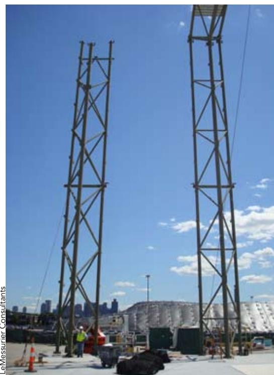
▲ The trussed frames were fixed to the foundation and self-stabilizing in all directions. Building end frames (left) were designed with additional bracing in between the tail pipes for additional torsional capacity.
