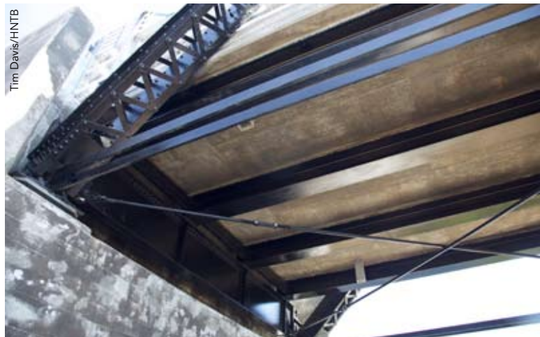
▲ At the bridge's new home on the Gateway Trail, a lightweight concrete deck is supported by new steel stringers.
