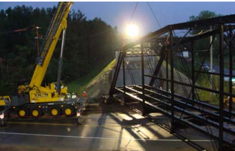
▲ In May 2011 two cranes lifted the truss and set it on its new abutments on the Gateway Trail.
