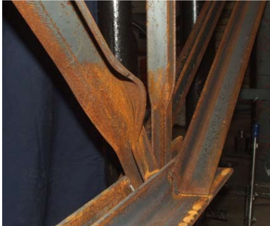
▲ Crimped angles and crimped angle local web buckling.
