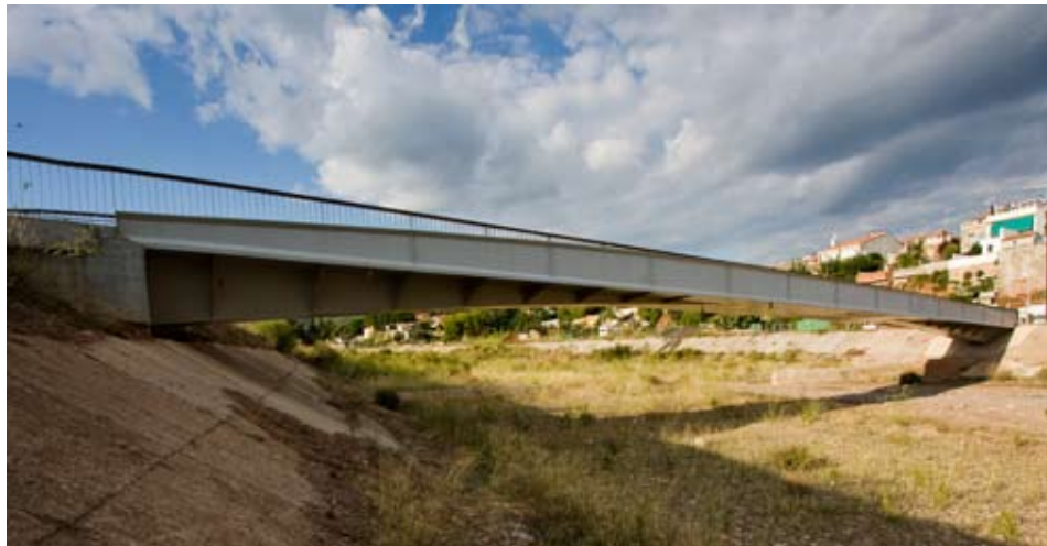
▲ Fig. 3. Matadapera pedestrian bridge.
