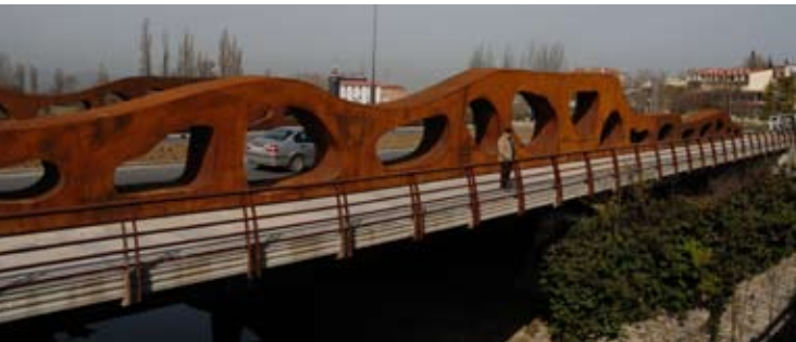
◀ Fig. 6. Abetxuko Bridge in Vitoria.
