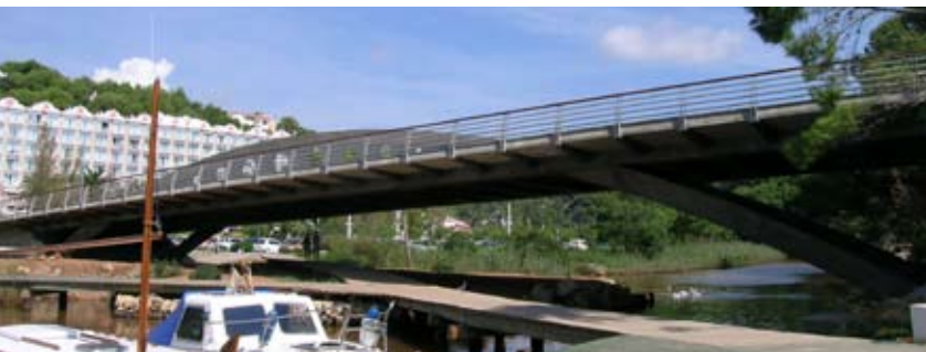
▲ Fig. 4. Stainless-steel road bridge in Minorca.
