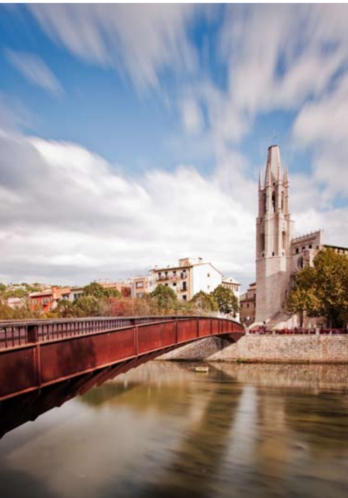
▲ Fig. 1. Girona pedestrian bridge.
