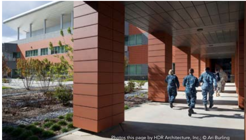
Photos this page by HDR Architecture, Inc., © Ari Burling
