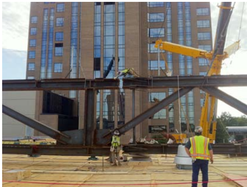
▲ Fig. 1: A two-piece truss being erected over an existing hospital building.
