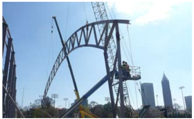
▲ Fig. 2: A multi-crane lift of a 226-ft-long barrel truss.
