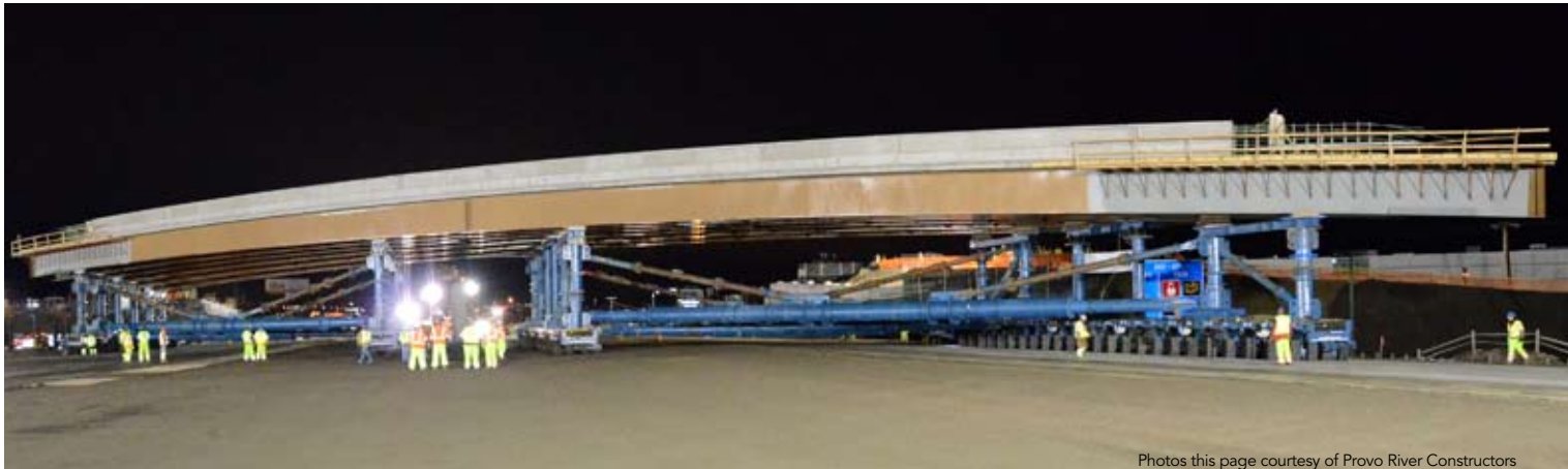
Photos this page courtesy of Provo River Constructors
