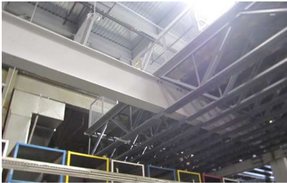
▲ Cantilevered joist framing at the mezzanine.
