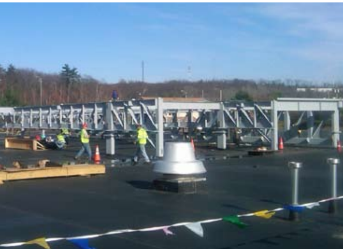
▲ Cantilevered joist framing at the mezzanine.
