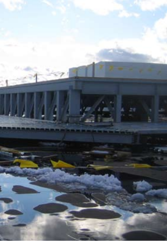
◀ Cantilevered snow shelf framing during construction as viewed from existing roof.
