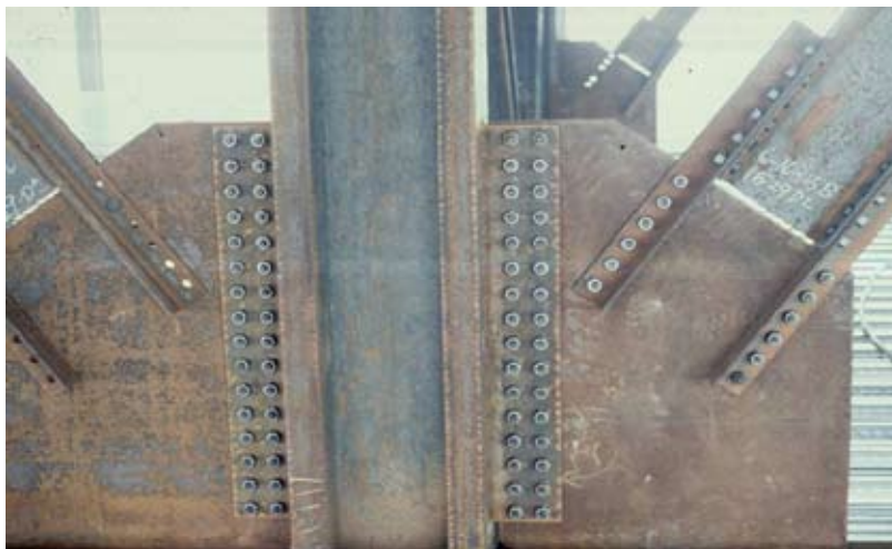
▲ A typical bolted brace connection.
