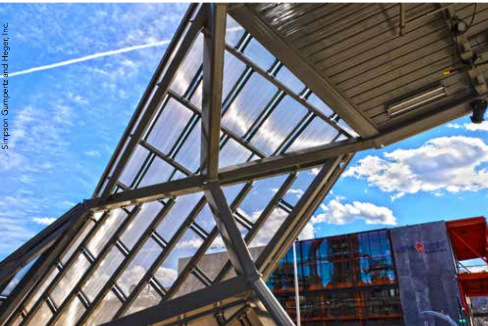
◀ The structure is a system of large support ribs, infill framing and secondary framing for exterior panels.
