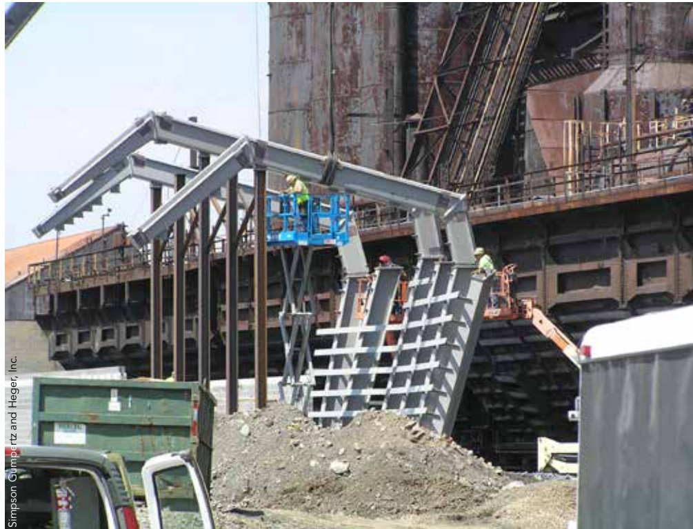
▲ Erection of the primary ribs, with shoring provided by temporary wide-flange columns.
