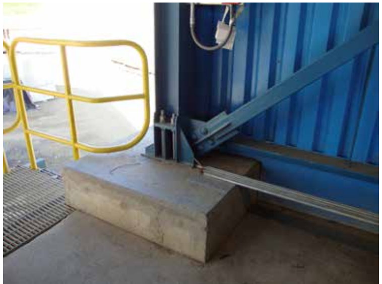
▲▼ Chilean braced frame anchorage details illustrating the provision of stretch length.
