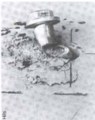
◀ Shear failure of a post-installed expansion anchor.
