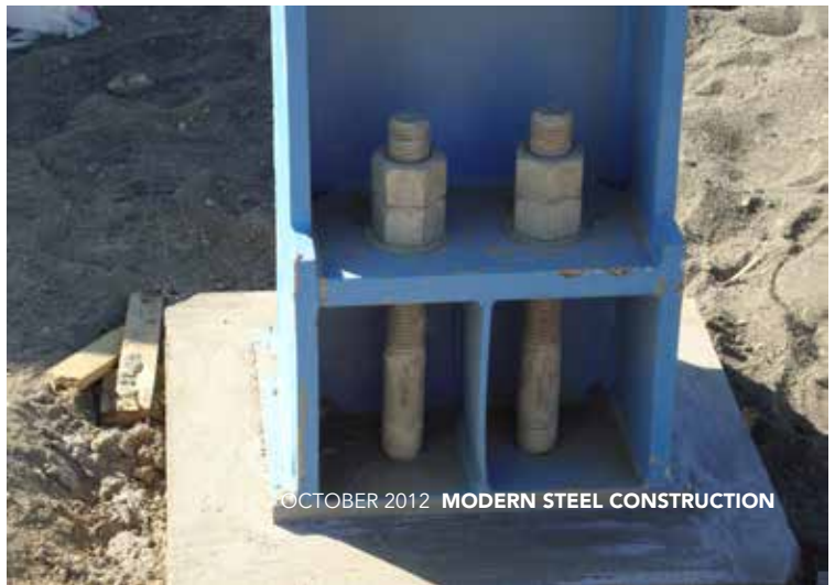
▲▼ Chilean braced frame anchorage details illustrating the provision of stretch length.
