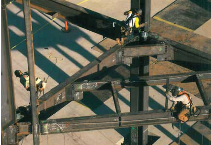
▲ Steel erection for the School of Engineering Library.
