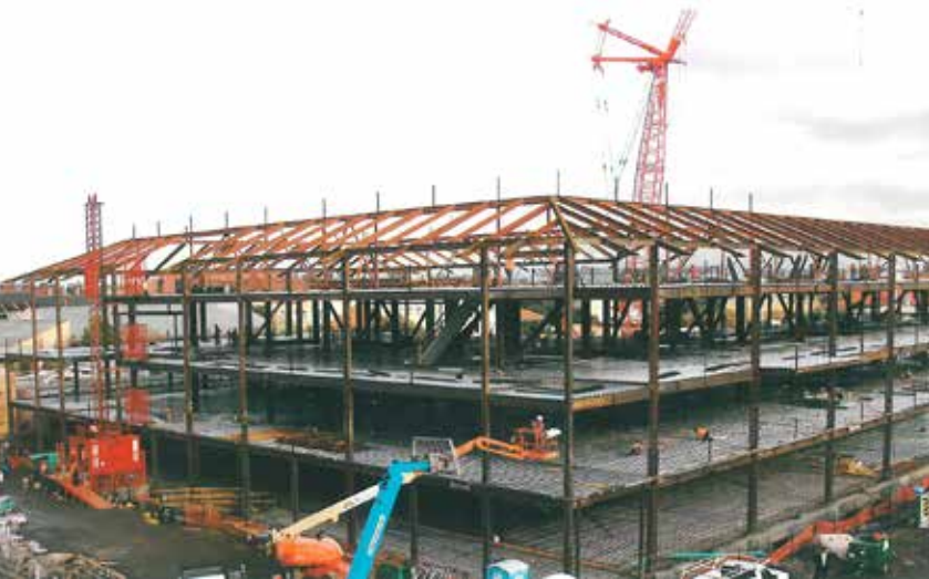
◀ Framing for the Environment and Energy Building, which used 1,470 tons of steel in all.
