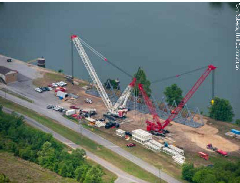
▲ The truss is assembled on the lakeshore...
