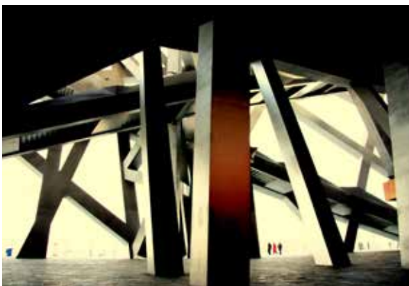
▲ The stadium is commonly known as “The Bird’s Nest” and is constructed with massive steel columns bended and arranged in an absolutely random pattern. In this picture, massive steel columns seem to fall out of the sky straight into the ground, raying in a random order. Standing in between them is like being in a natural crystal cave, an amazing spatial experience. The three people in the background provide a perspective of the size of these steel columns. —Xiaolong Li
