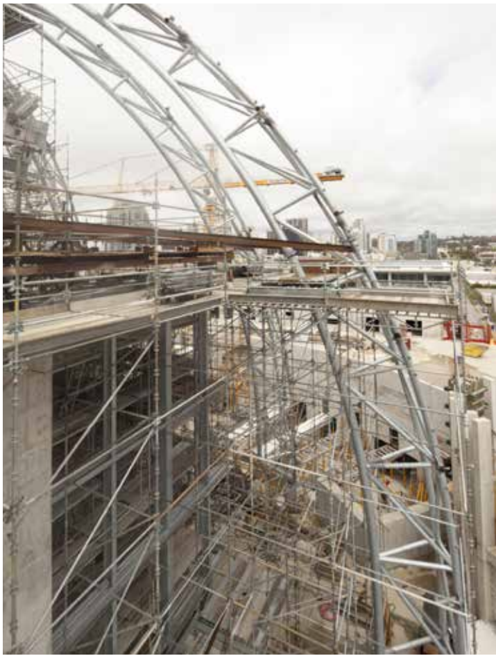
▲ The steel dome uses 285 tons of HSS in all. The largest steel sail measures 123 ft high by 53 ft wide.
