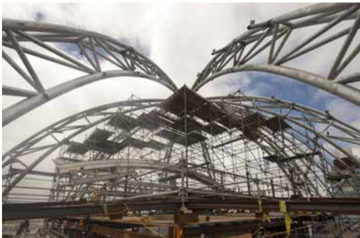
▲ The steel dome uses 285 tons of HSS in all. The largest steel sail measures 123 ft high by 53 ft wide.
