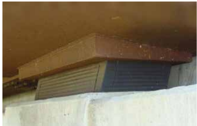
▲ Elastomeric bearings are typically detailed with rectangular shapes, which provide the most cost-effective solution.
