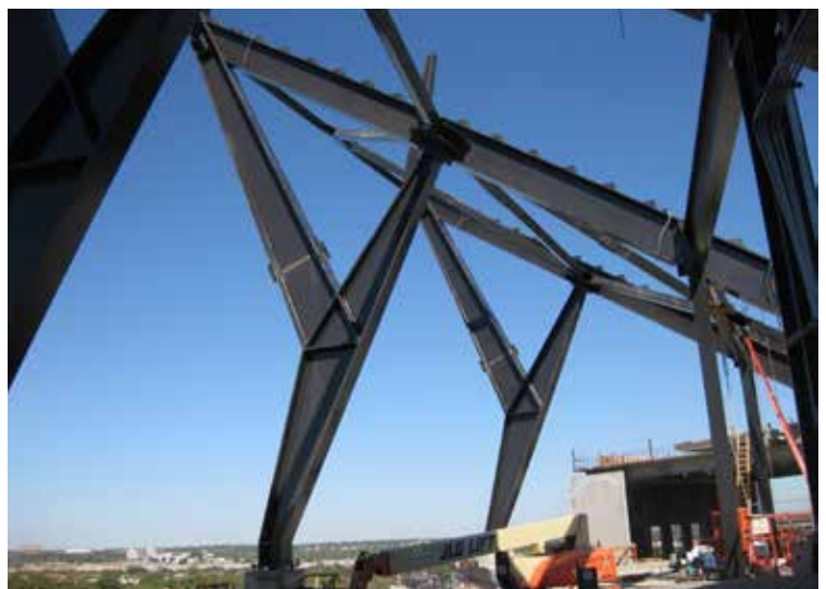
▼ "Y" column during erection of the northwest expansion.
