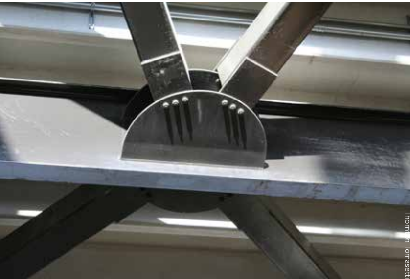
▲ Inclined bracing connection at the upper seating level.
