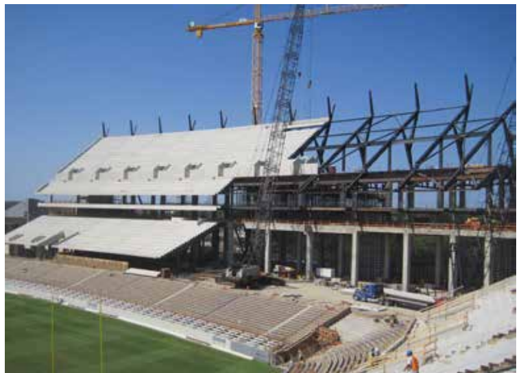
▲ West stands during erection.
