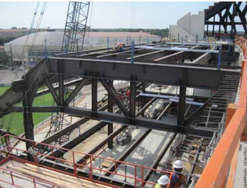
▲ Truss at the Upper Concourse during erection.
