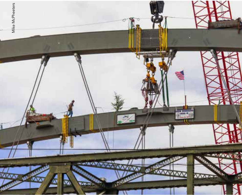
▲ The final arch rib, in place.
