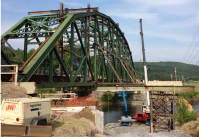
▼ Erecting the new steel. Approximately 120 tons were added.
