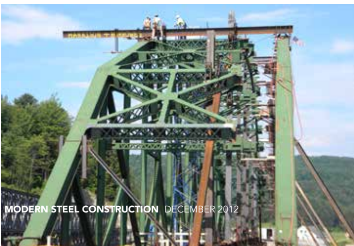
◀ A team of 25 people from the design-build team were all on-site the day of the big move to carefully monitor 10 critical connection points that, when cut free, would expose the truss to potential distortion and twisting.
