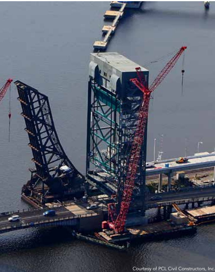
Courtesy of PCL Civil Constructors, Inc.
